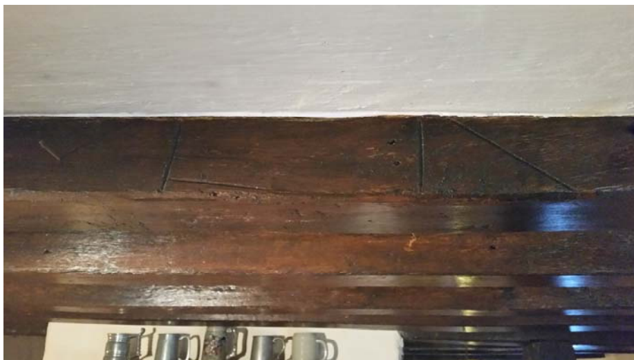
Beams inside the adjoining cottage
