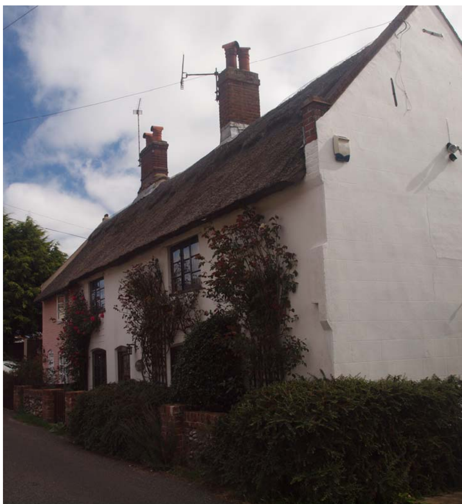
The three adjoining cottages (now two)
